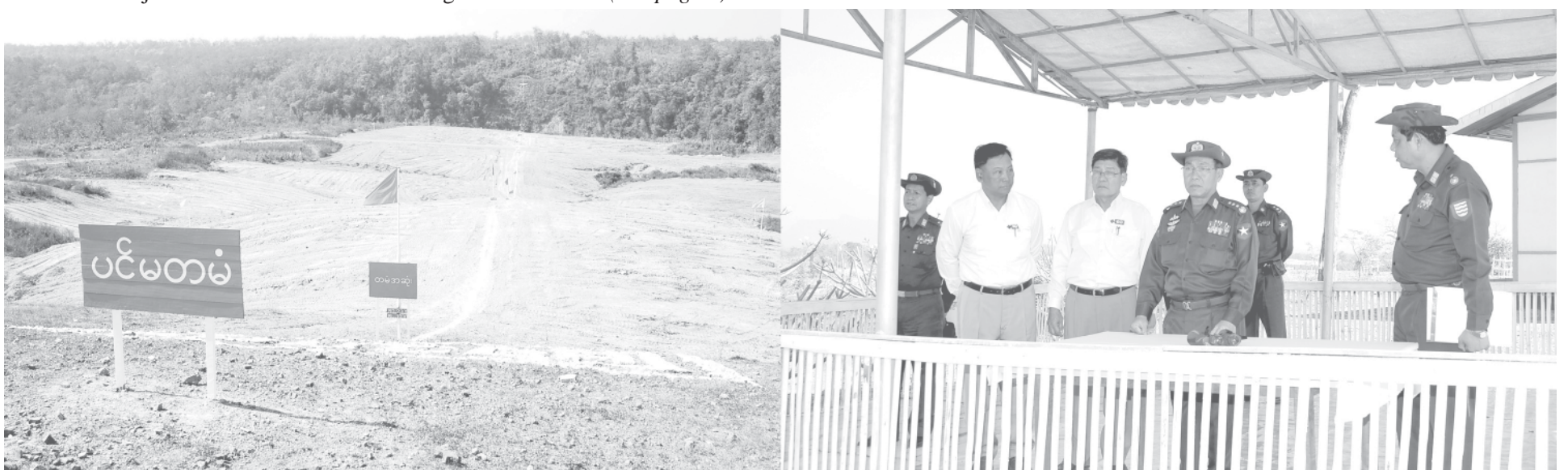
Prime Minister General Soe Win inspects construction of Myittha River Multi-purpose Dam. — MNA
