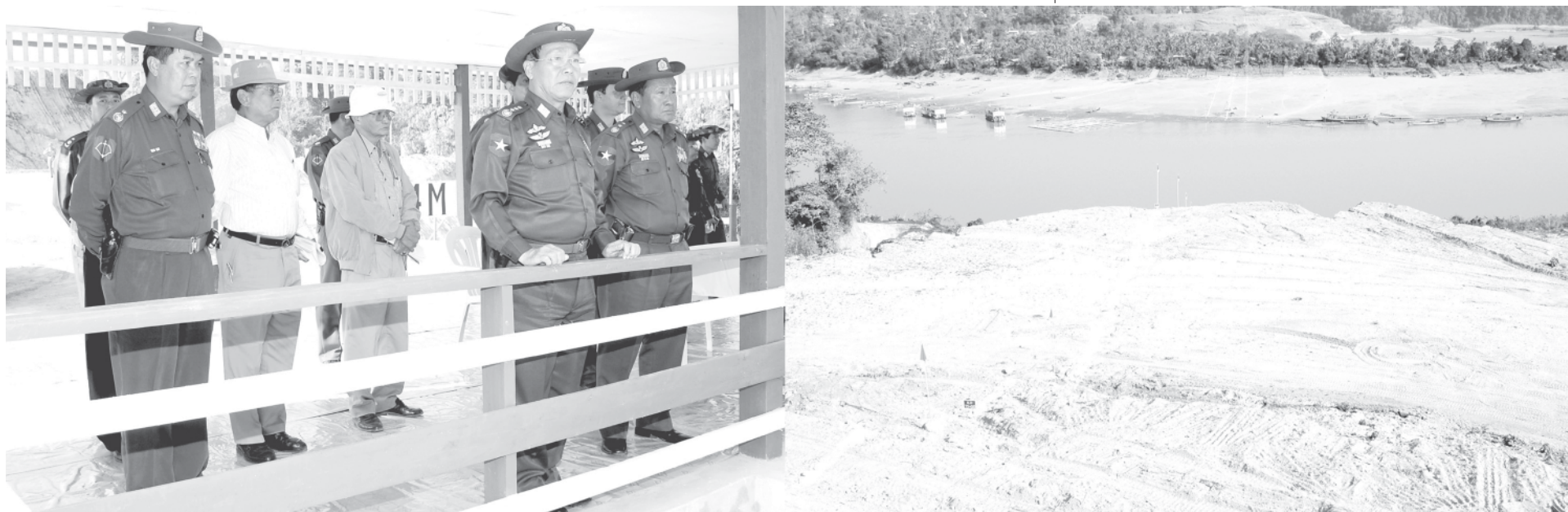
Prime Minister General Soe Win views construction work of Htamanthi Dam and Hydroelectric Power Multipurpose Project.—MNA
