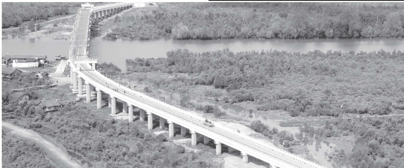
Aerial view of Minkyaung Creek Bridge in Rakhine State, a symbol of the government's goodwill to bridge the development gap. — MNA
