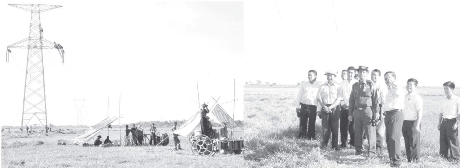
Maj-Gen Khin Maung Myint inspects construction of Hlinethaya-Yekyi (Athoke) power line in Nyaungdon Township. — MNA
