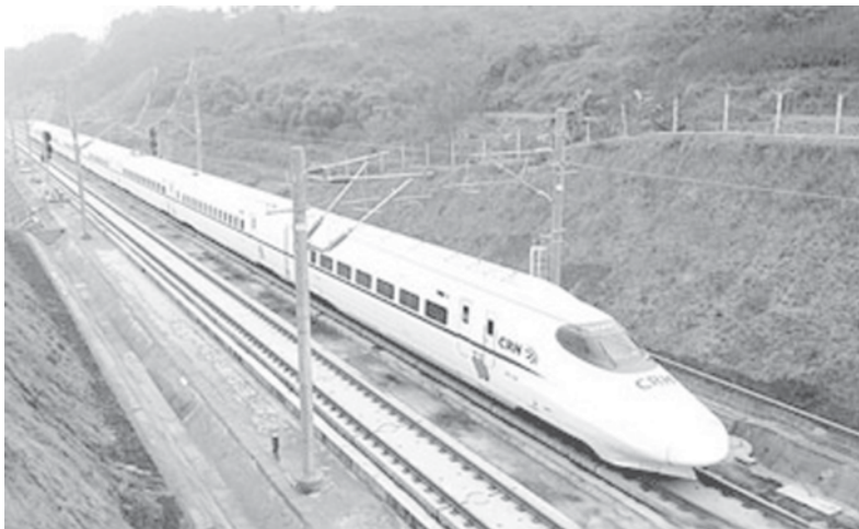
China has successfully conducted an operational test on its first domestically developed, concrete-bed rail track, with high-speed trains in southwest China.— XINHUA
