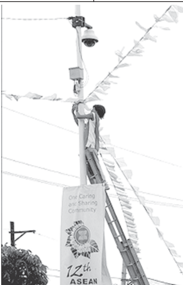
A worker decorates a lamp post equipped with a security camera outside the Cebu International Convention Centre as part of security for the Association of Southeast Asian Nations (ASEAN) Summit and East Asia Summit recently.—INTERNET
