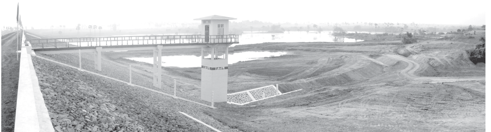
Hlaing Chaung Dam in Pale Township. — AGRICULTURE AND IRRIGATION
