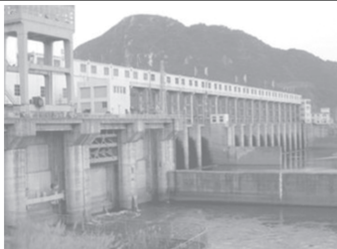
Baishiyao Dam on the North River is seen in this picture taken in Yingde, south China's Guangdong Province, on 22 Dec, 2005.
