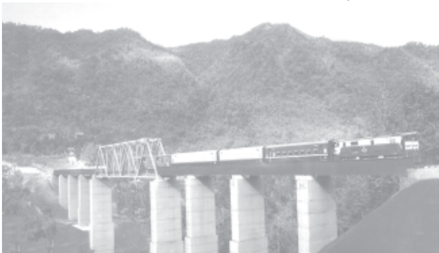
A train passes over Pon Creek Bridge on Taunggyi-Saikkhaung-Namhsan Railroad.
