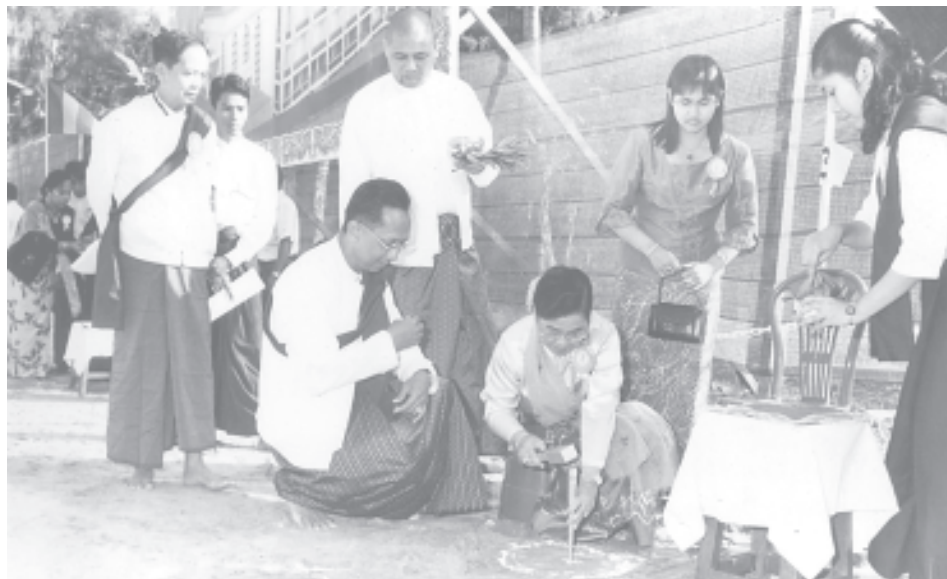
Daw Khin Than Nwe, wife of Lt-Gen Tin Oo, drives a stake for construction of Dhammayon of Mahasi Sasana Yeiktha.— MNA
