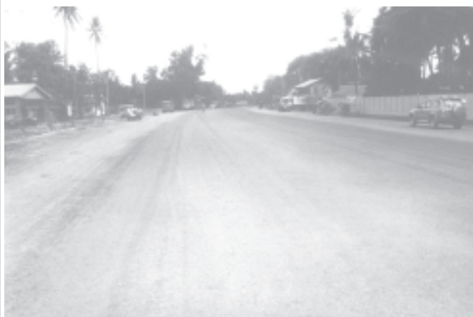
Progress in upgrading Mandalay-Meiktila section of Yangon-Mandalay Six-lane Highway.
