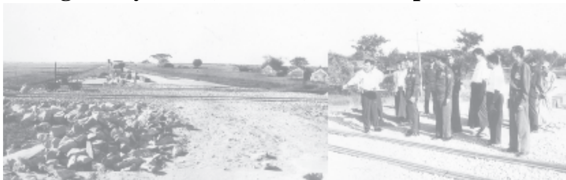
Commander Lt-Gen Myint Swe inspects Inwa Road linking Dagon Myothit (South) and (East) townships and construction of level crossing on crossing road Yangon-Mandalay Rail Road. —MNA
