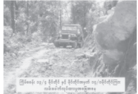
Construction work between 13/4 mile post and 14/0 mile post
