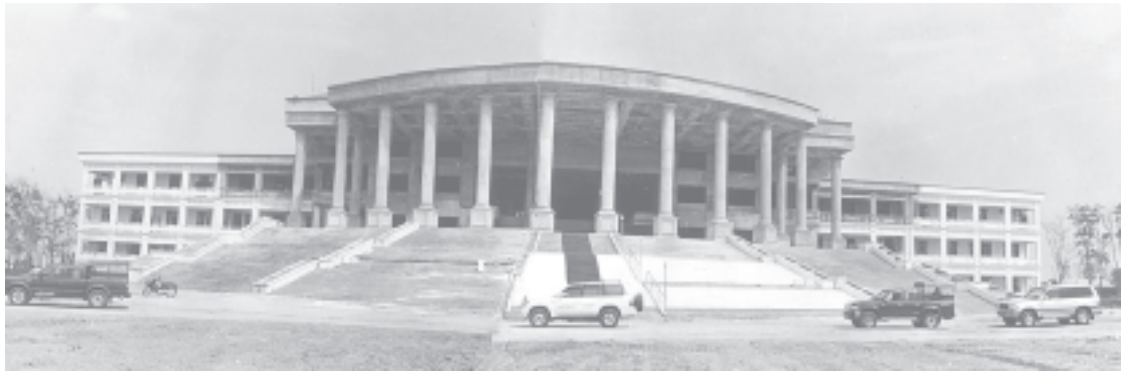
Construction of Myeik University in progress.—MNA
