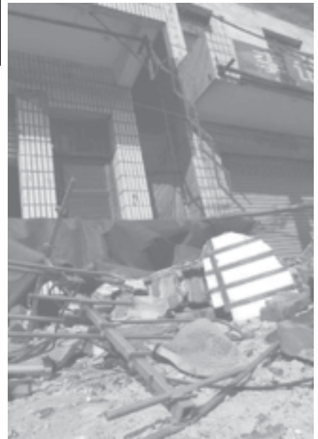
Debris is seen at a street in Gangkou township of Jiujiang County, east China's Jiangxi Province, on 26 Nov, 2005.—INTERNET
