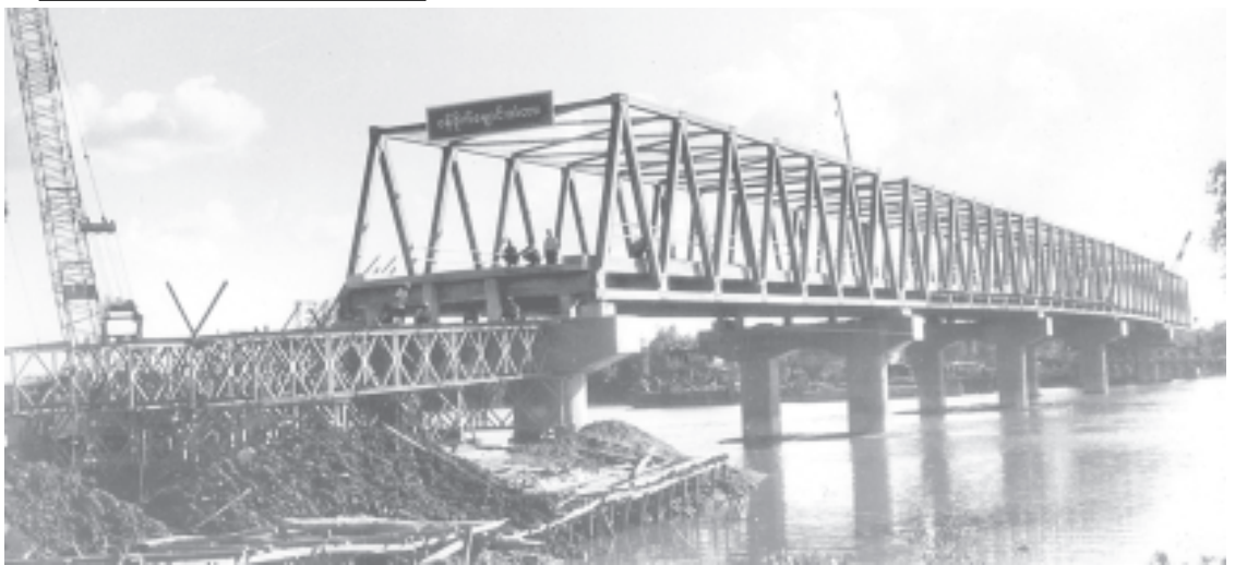
Wunphaik Bridge being built in Yanbye Township. — MNA
