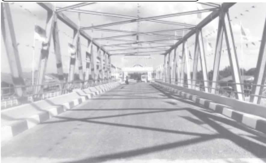
Thanthamachay Bridge on Yangon-Kyaukpyu Road in progress. — MNA
