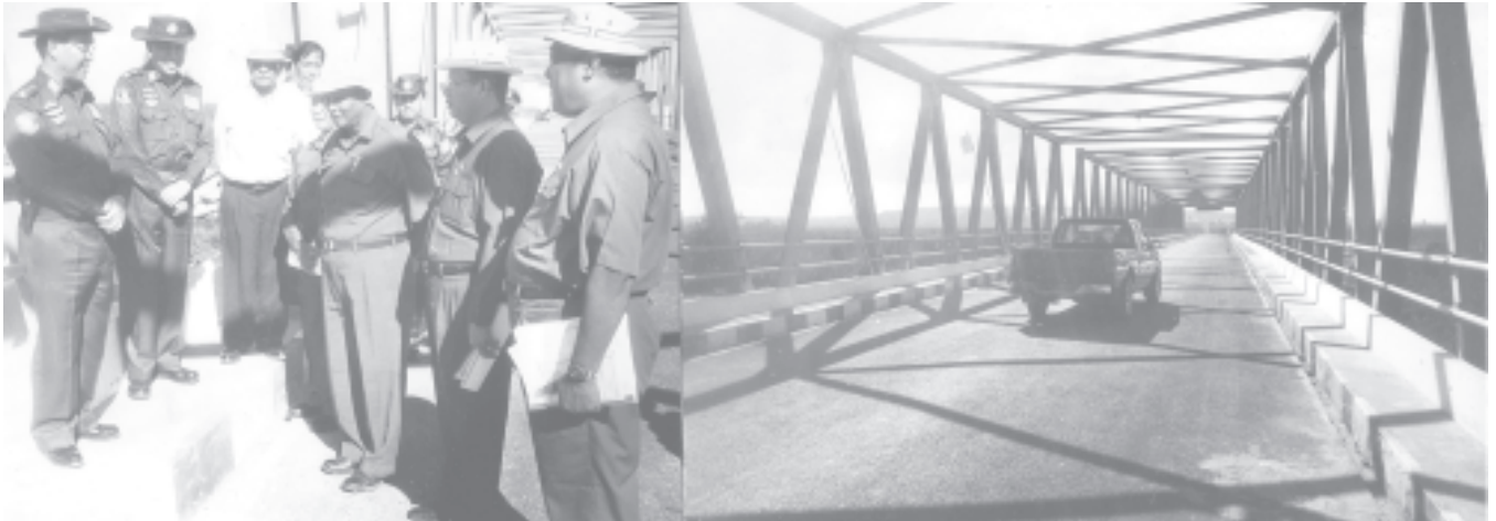
Prime Minister General Soe Win inspects construction of Minkyaung Creek Bridge in Yanbye Township. — MNA
