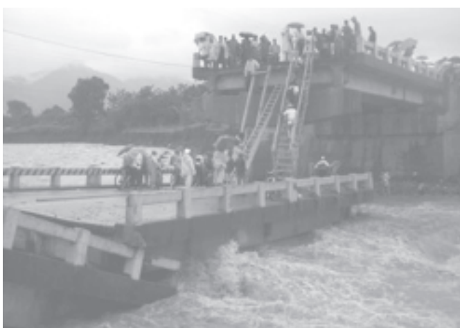
Residents try to cross a bridge over the Monga River in Saba, northern Honduras, which collapsed because of the heavy rains on 18 Nov, 2005. Tropical Storm Gamma formed Friday off the coast of Honduras, the 24th named storm of an already record-breaking Atlantic hurricane season.—INTERNET
