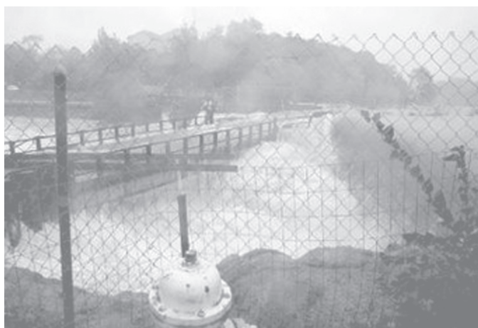
The flooding Ramapo River roars over a dam under reconstruction in Pompton Lakes, New Jersey, on 14 October, 2005.
