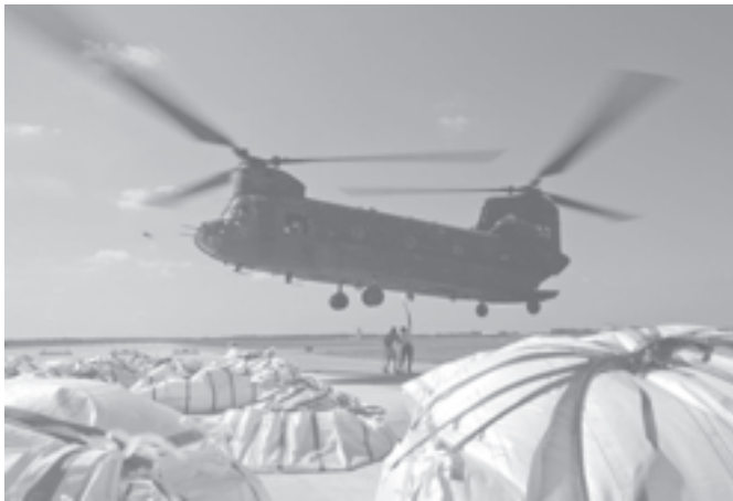
Antonio Smith (L) and Clarence Bonvillain hook up a 6 to 7 thousand pound (2722-3175 kg) sand bag to a military helicopter at the Houma airport in Louisiana on 27 September, 2005. The Army Corps of Engineers used helicopters in an attempt to shore up a flood wall breach at the Montegut levee, caused by Hurricane Rita, where a tidal surge caused more flooding to an already damaged area. — INTERNET
