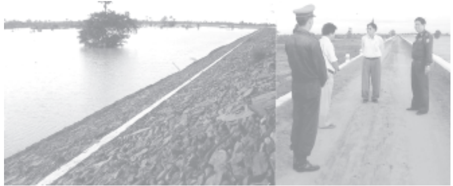
Maj-Gen Htay Oo inspects Nyaungon Dam being built in Meiktila Township. A&I
