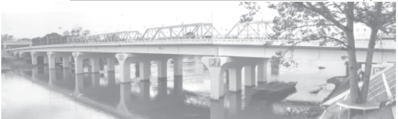
Newly-built Myingte Bridge lies on Yangon-Mandalay Six-lane Union Highway between Singaing and Amarapura Townships.— MNA
