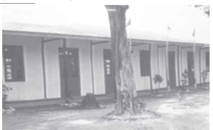
The new 120' x 30' four-unit building of Basic Education High School in Natgyichaung Village, Paung Township, Mon State. — MNA
