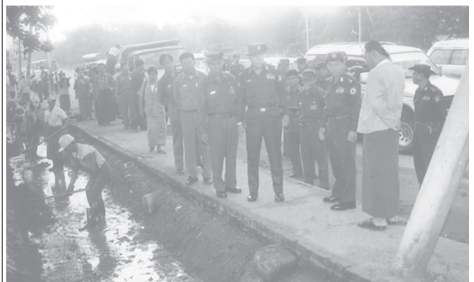
Commander Maj-Gen Myint Swe and Mayor Brig-Gen Aung Thein Lin inspect dredging of the drain at Sawbwagiyon Junction in Insein Township.—MNA
