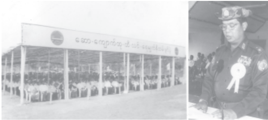
Commander Maj-Gen Tha Aye addresses the opening of Saw-Kyaukhtu-Htilin-Yaymyetni road. — CONSTRUCTION
