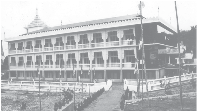
Newly built Myittavihari three-storey Dhammayon of Hpa-uk Tawya Buddha Sasana Yeiktha (Main) in Mawlamyine.—MNA
