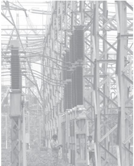
Indonesian employees of the state electricity company check a power grid located on the outskirts of Jakarta on 18 August, 2005.
