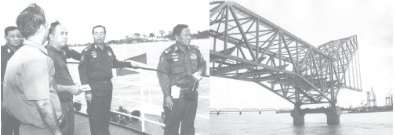
Prime Minister General Soe Win inspects Ayeyawady Bridge (Yadanabon) Project on Mandalay bank. — MNA
