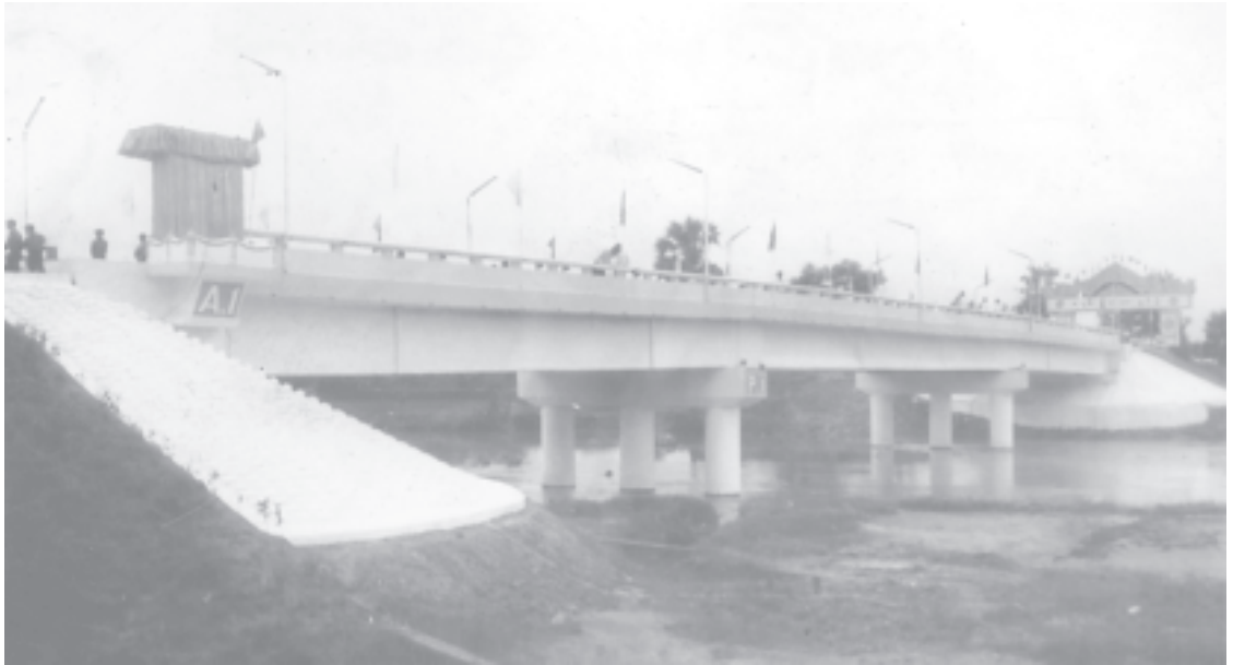
Mayanggu Bridge in Einme Township, Myaungmya District, Ayeyawady Division. — CONSTRUCTION
