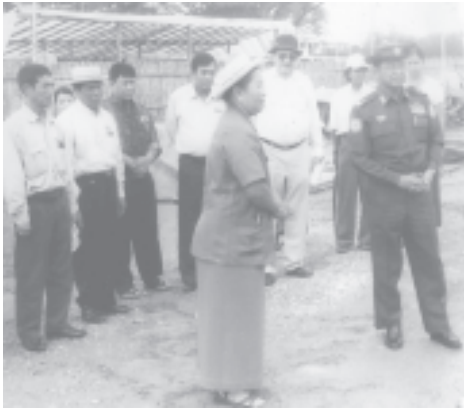
Minister Maj-Gen Saw Tun inspects construction of Panmawady Bridge (Myintkaseik) in Ayeyawady Division. — CONSTRUCTION
