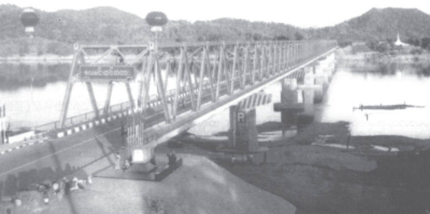
Bala Min Htin Bridge across Ayeyawady River. — MNA
