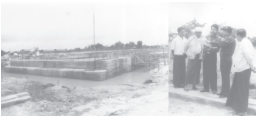
Minister Maj-Gen Saw Tun inspects Twantay Bridge construction site. — CONSTRUCTION
