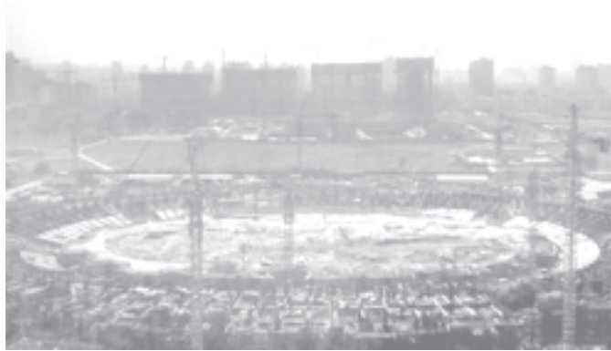
Construction is underway for the Olympic stadium in Beijing on 30 June, 2005.
