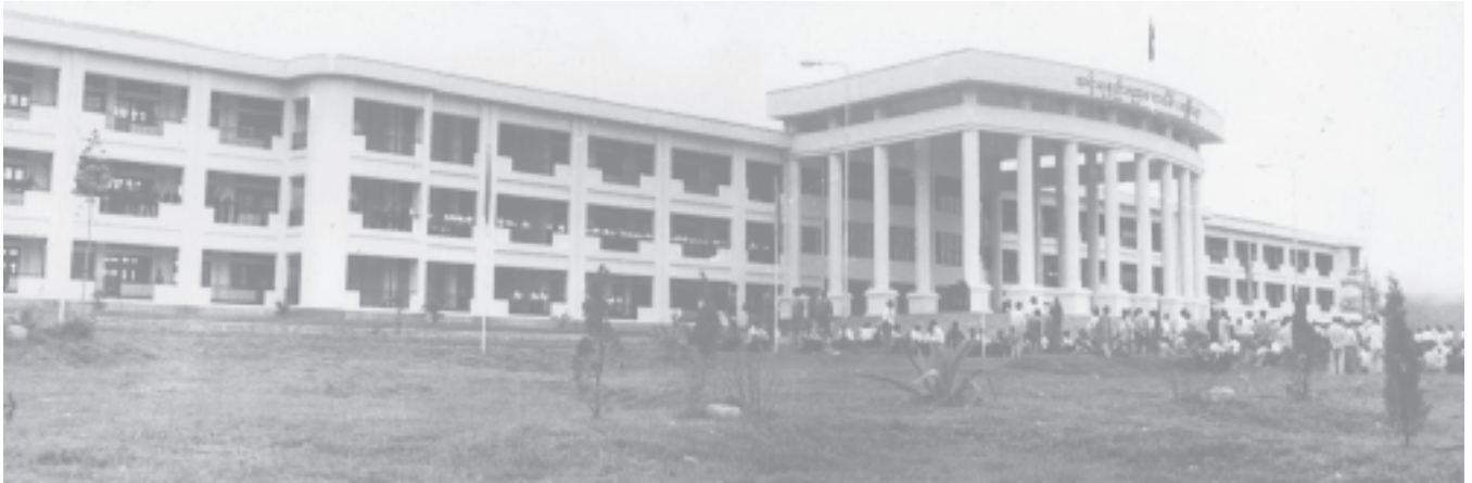
Main building of Government Technological College (Kengtung) —MNA
