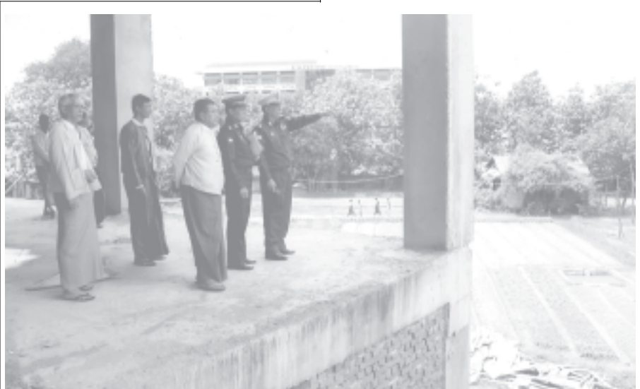
Minister for Culture Maj-Gen Kyi Aung, Deputy Minister Brig-Gen Soe Win Maung view the construction site of new National Library. — CULTURE
