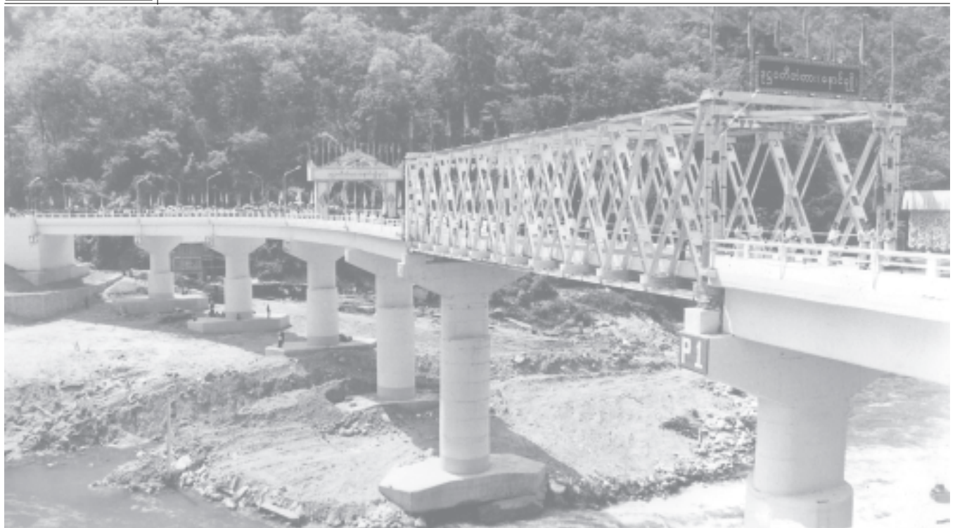
Dokhtawady Bridge (Nawngkhio) linking Yaksawk Township of Shan State (South) and Nawngkhio Township of Shan State (North) was commissioned into service on 6 June 2005. — MNA
