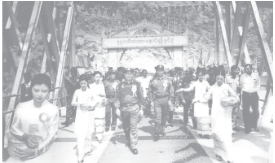
Prime Minister Lt-Gen Soe Win and party inspect Dokhtawady bridge. — MNA
