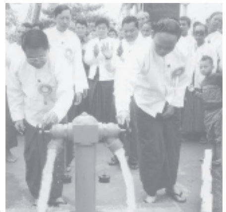
Mayor Brig-Gen Aung Thein Lin and Vice-Mayor Col Maung Pa put Ngamoeyek Gyobu pipe into service.— YCDC
