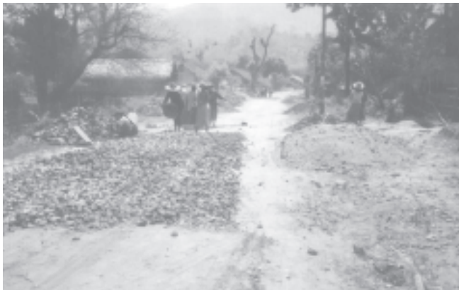
Dophonyan-Theinlon gravel road being constructed.
