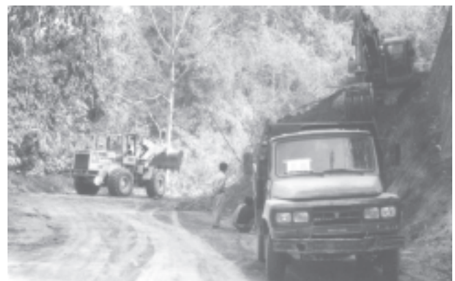
Myitkyina-Bhamo road being upgraded with the use of heavy machinery.
