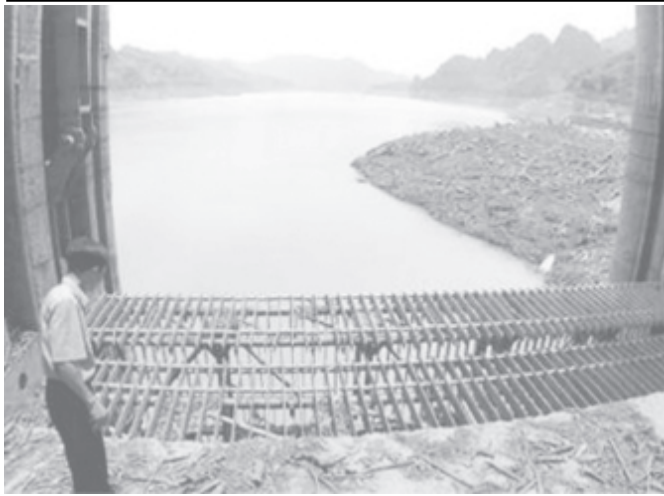
A Vietnamese engineer visits a dam in Vietnam's biggest Hoa Binh hydro power plant in the northwest Hoa Binh Province on 25 May, 2005.
