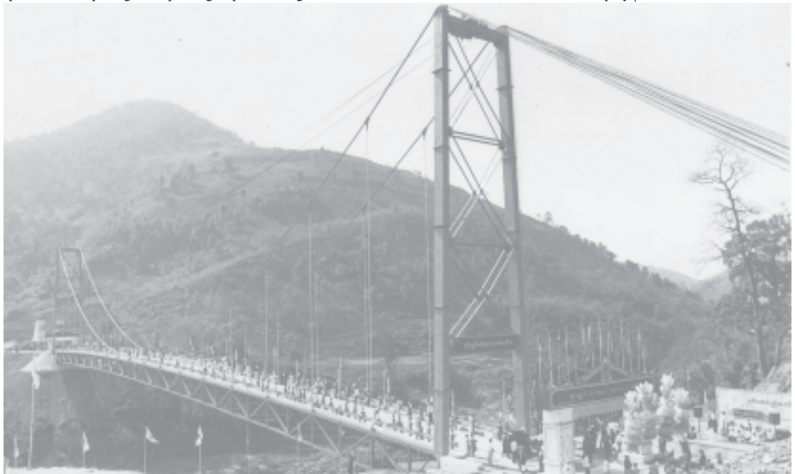
Newly commissioned Thanlwin Bridge (Tapar) built in Kutkai Township of Muse District. — MNA
