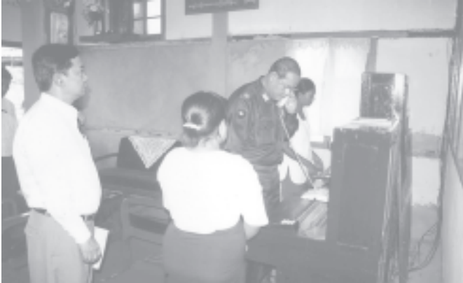
Minister Brig-Gen Thein Zaw inspects the telephone exchange in Wakema on 14-5-2005. —COMMUNICATION
