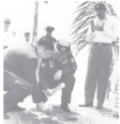
Prime Minister Lt-Gen Soe Win drives the stake to build 50-ton quality paper plant. — MNA
