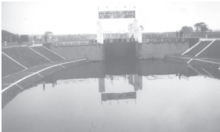
The gate of Kayan Sluice Gate for vessels. — MNA
