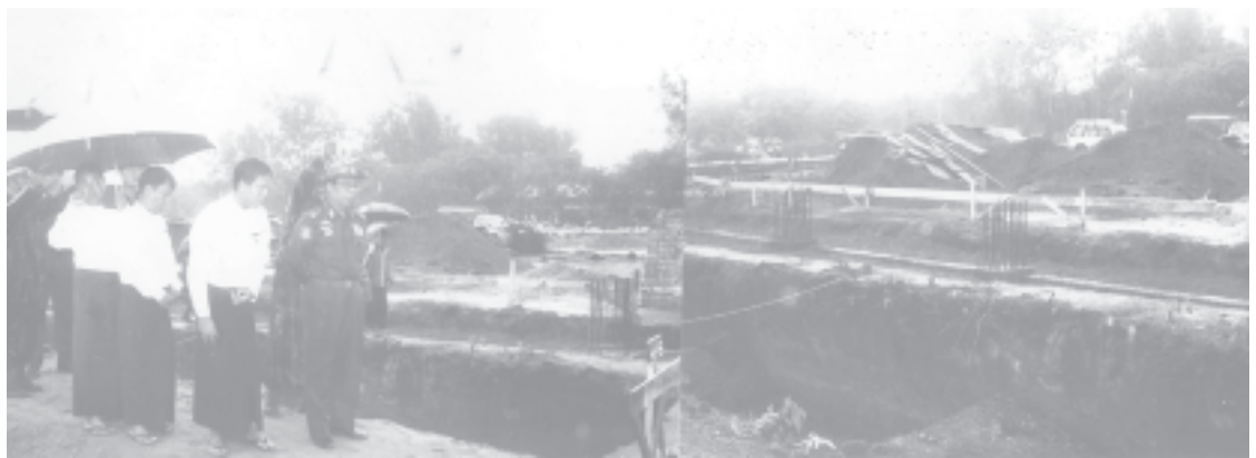
Lt-Gen Maung Bo views the site chosen for construction of the three-storey building of GTC (Mawlamyine). — MNA
