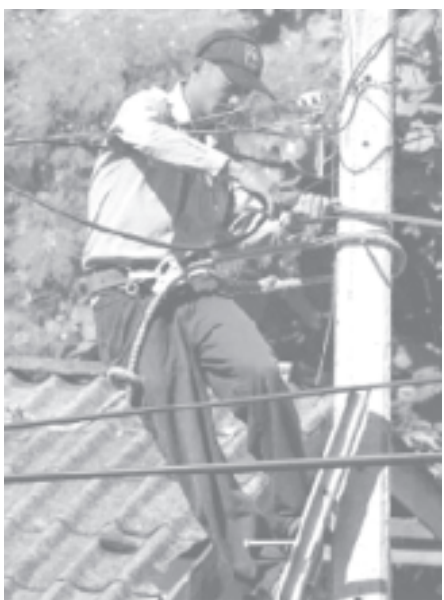
A worker fixes electricity cables in Vientiane on 7 May, 2005.
