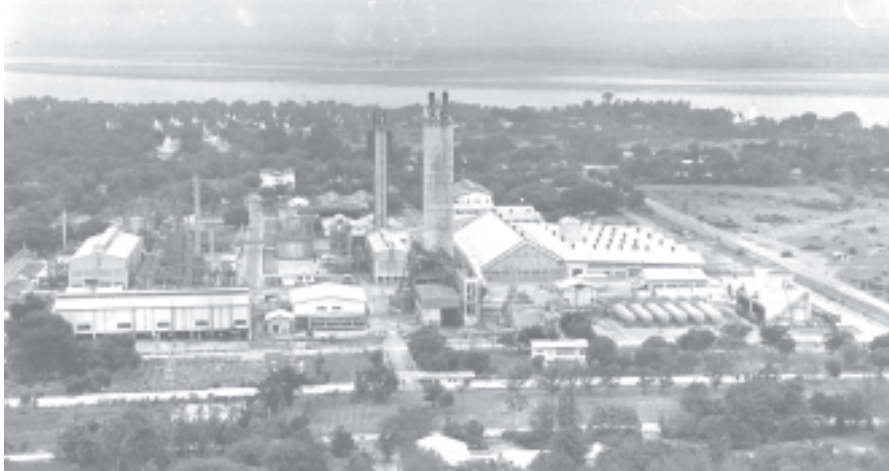
Aerial view of No 1 Fertilizer Plant (Sale) of Myanma Petrochemical Enterprise in Chauk Township.— MNA
