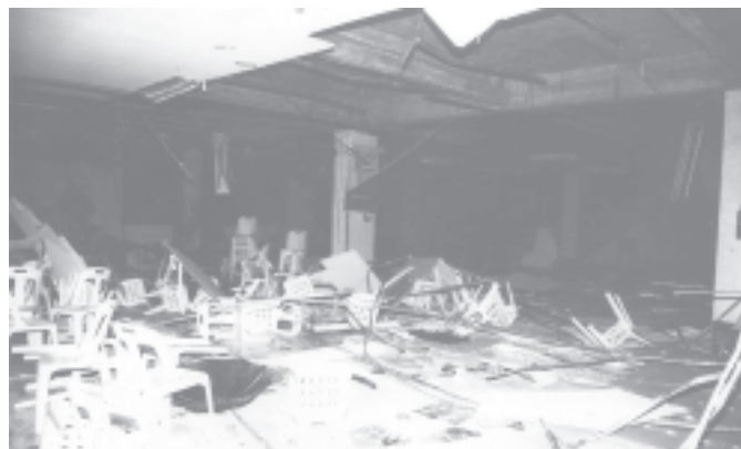
Damages at Yangon Trade Centre in Pazundaung Township where a time bomb was exploded.— MNA
