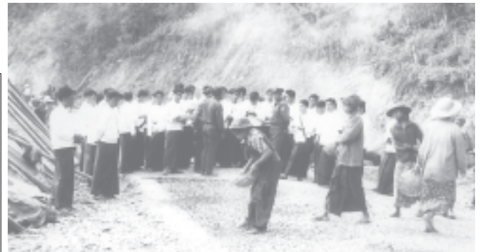
USDA members view road construction in Mindat.— MNA
