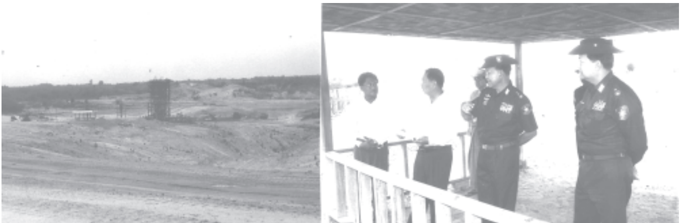
Lt-Gen Khin Maung Than inspects construction site of Wagadok Dam Project near Taunghsat-in Village in Bago Township, Bago Division. — MNA
