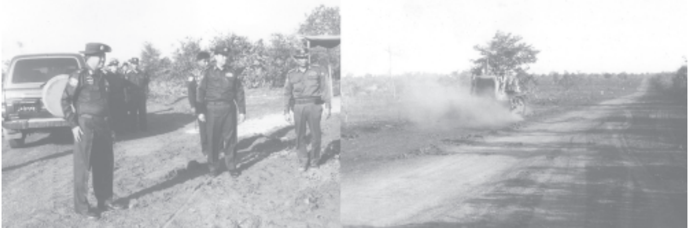
Lt-Gen Khin Maung Than inspects extension of 25 miles and 6 furlongs long road linking Kyonmaku Creek and Shwegyin.— MNA
