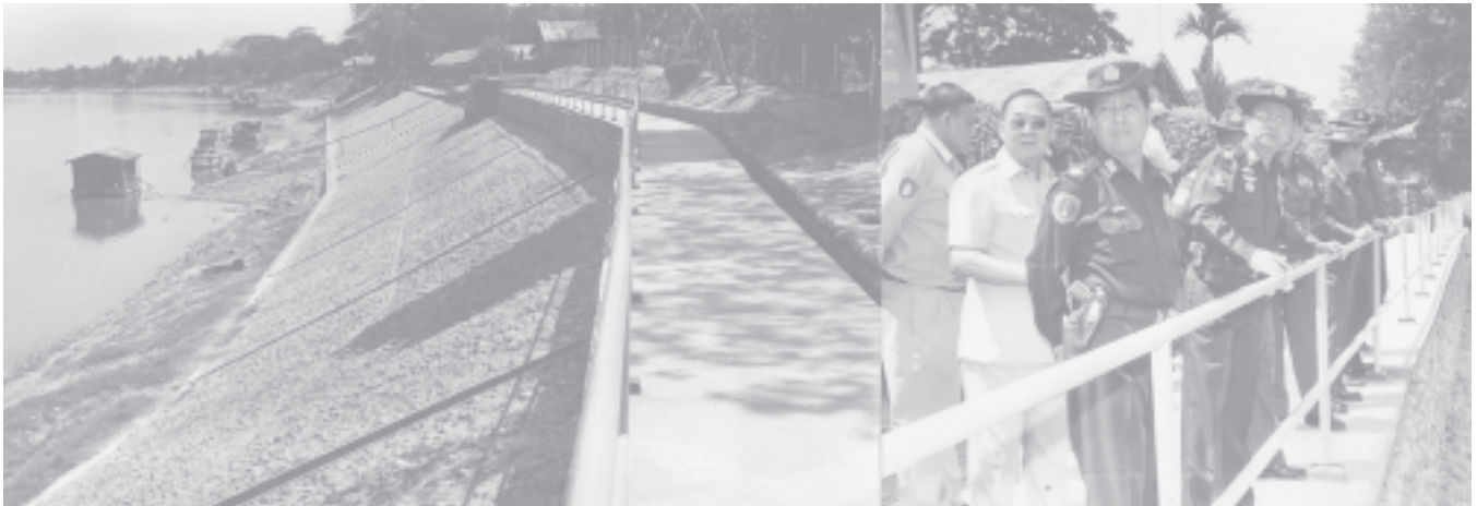
Secretary-1 Lt-Gen Thein Sein inspects progress of building retaining walls at Ayeyawady River in Myitkyina.— MNA
