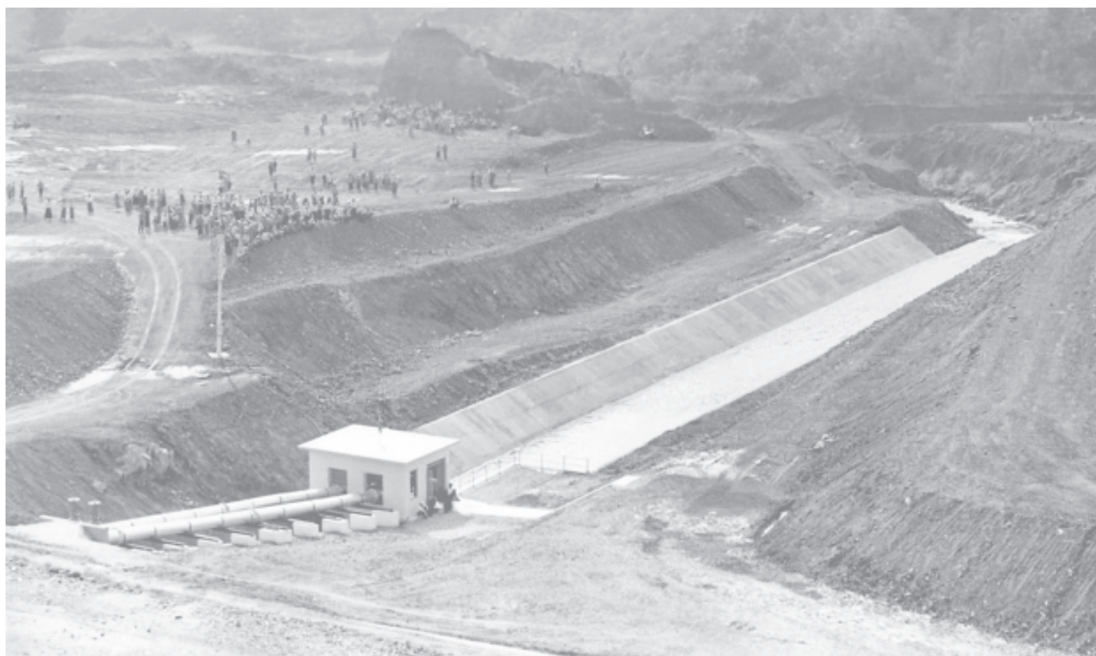
Aerial view of conduits at Kunchaung Dam. — MNA
