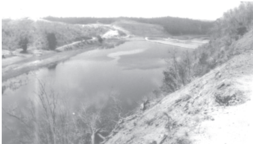
Kyeewon Kyeewa Multi-purpose Dam Project on Mone Creek in Pwintbyu Township, Magway Division.
