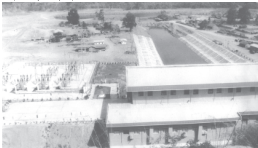
Monechaung Hydel-power Plant that generates 75 megawatts.
