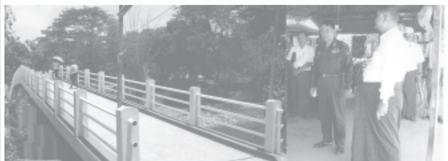
Minister Brig-Gen Maung Maug Thein inspects a concrete bridge in Kayan Township. —MNA
